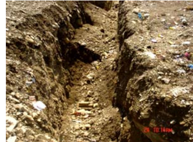
Figure 3.4.2 Pre-Excavated for Disposal of Solid Waste
