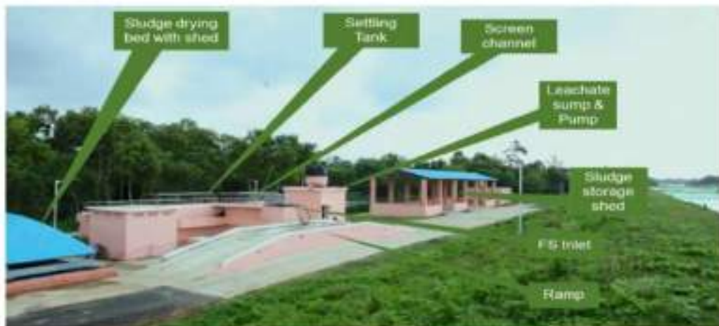
Figure a: STP-cum-FSTP to treat sewage and faecal sludge in the same facility
